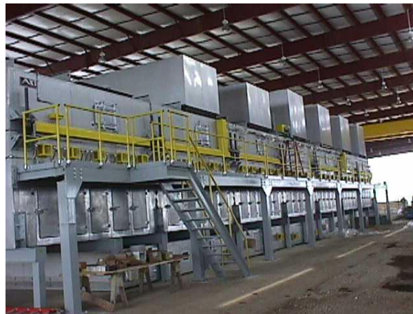
Figure 2. Seven-zone, glass mat thru-air dryer during installation
