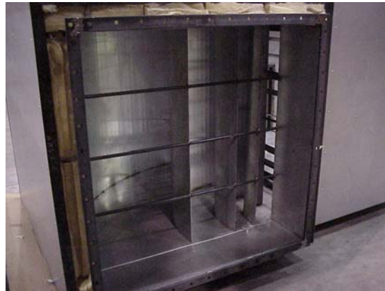
Figure 4. In-duct splitter vanes
